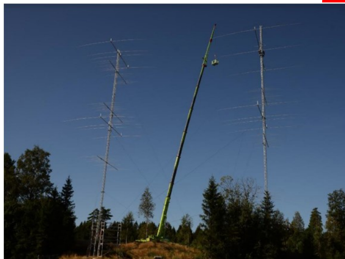
Figure 2 The two 56-meter towers, and E77DX installing the 80m beam.
