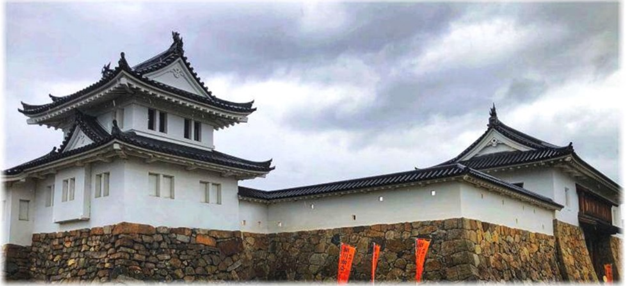
Main buildings that remain of Tanabe castle
