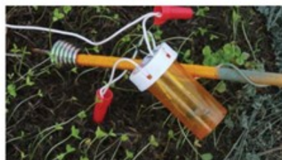
Above is the schematic for the termination end of the beverage. The picture shows one actually installed. Another "pill bottle" is used here. Note the wire nuts making the connections.
