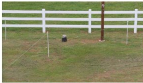
Here are three Beverages (in different directions) coming to a common feed point. A plastic "bucket" makes a weather-proof cover for the three Beverage feedpoint.
