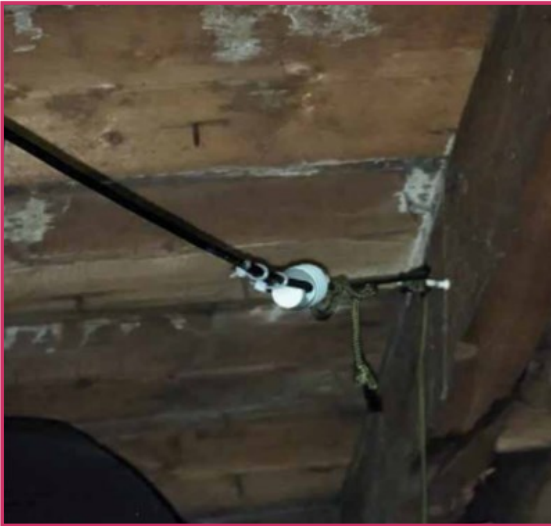
The end of one of the dipole elements tied onto a cup hook screwed into one of the roof timbers.
